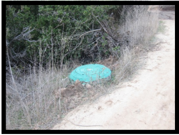
12. Manhole #48 Left of the path, North of Balboa Ave.
