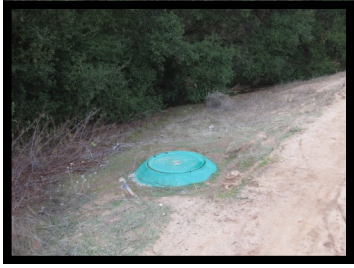
11. Manhole #49 Just left of path, North of Balboa Ave.
