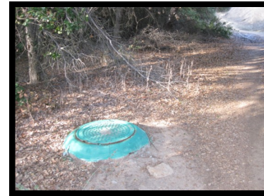
17. Manhole #305 Just left of the path, North of Balboa Ave.
