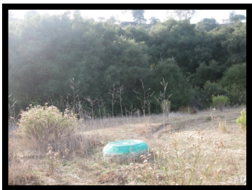
14. Manhole #70 10' left of the path, North of Balboa Ave.
