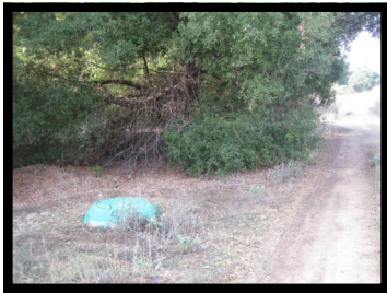
13. Manhole #66 5' left of the path, North of Balboa Ave.
