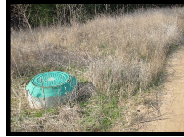
16. Manhole #304 Just left of the path, North of Balboa Ave.
