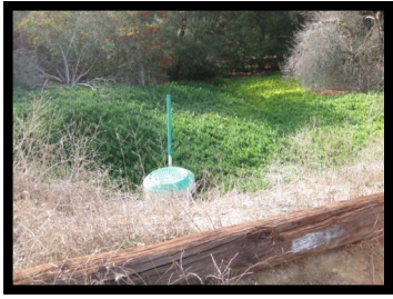
10. Manhole #47 15' left of path at beginning of trailhead, North of Balboa Ave.
