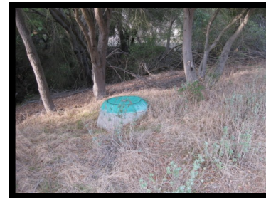
18. Manhole #306 10' left of the path, North of Balboa Ave.
