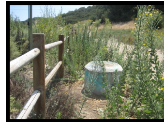
16. Manhole #191 N 32° 50' 44", W 117° 11' 12"
