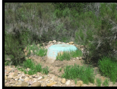
24. Manhole #163 N32.788942 N W117.135570
