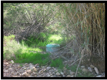
27. Manhole #46 N32.791138 N W117.136486
