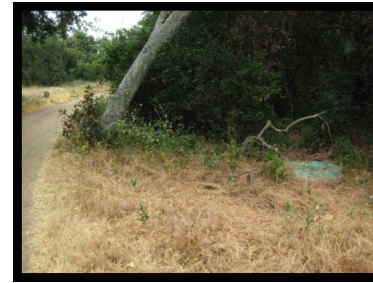
15. Manhole #1 32° 56' 13" N 117° 08' 47" W
