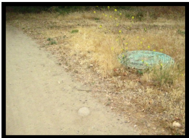
13. Manhole #3 32° 56' 12" N 117° 08' 36" W
