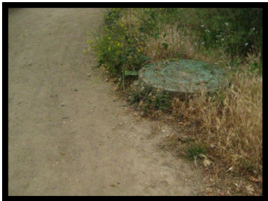
12. Manhole #4 32° 56' 11" N 117° 08' 33" W
