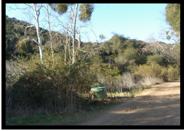
11. Manhole #5 32° 56' 12" N 117° 08' 30" W
